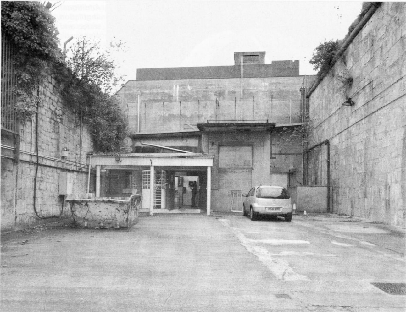
The inner court yard at the end of the dry ditch and the entrance into the Maritime Headquarters.
